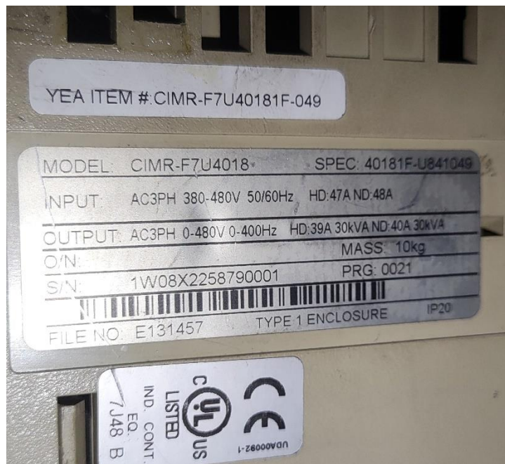
Gambar 6. Nameplate Variable Speed Drive Yaskawa
