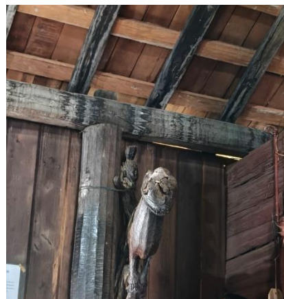
Image of columns and beams on the wall
